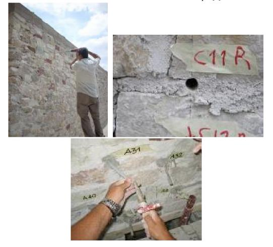
Figure 5. Grout injection procedure, drilling holes in mortar joints and fixing
