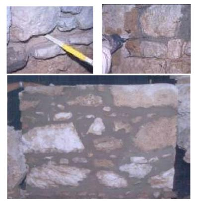
Figure 1. Grout injection procedure, drilling holes in mortar joints and fixing
