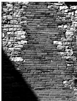
Figure 9. Masonry replacement intervention
