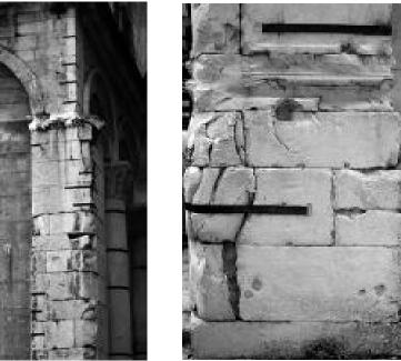
Figure 2. Crack fastening by metal bars
